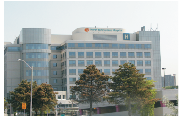
North York General Hospital, Toronto, Ontario
